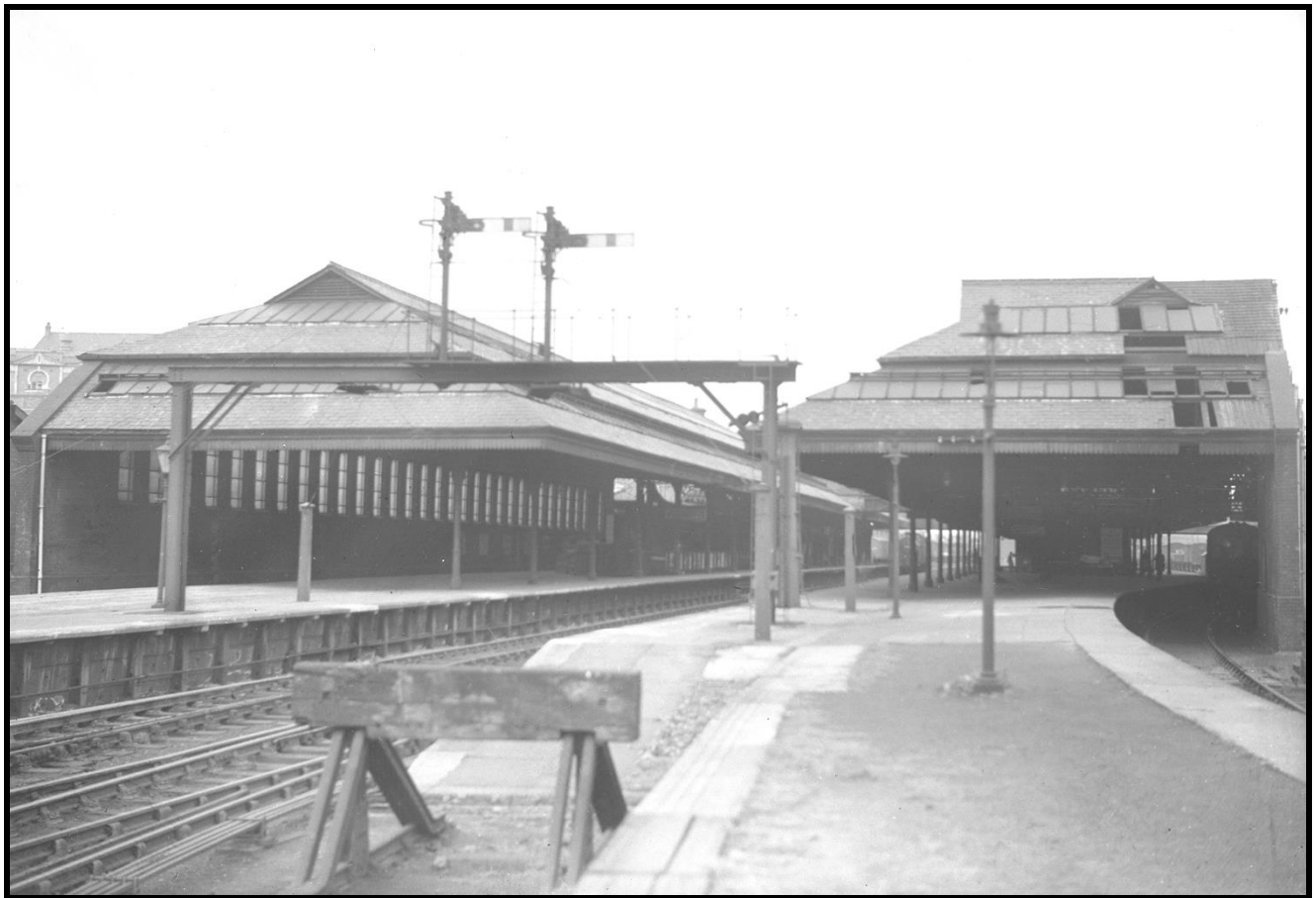
St Helens Shaw Street station, 1951 (66312)
