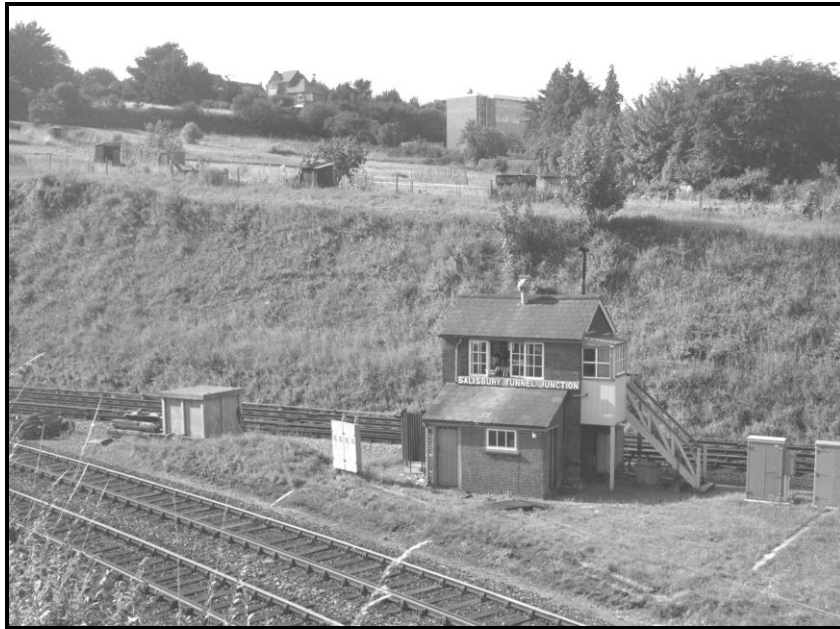
Salisbury, Tunnel Junction signal box in 1960s (39499)
